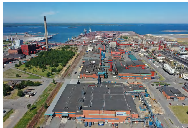
Site van Rechargeable Battery Materials in Kokkola (Finland)
